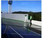
The solar roof was installed to distribute electricity at the headquarters in Bangkhen area on 12 January 2023, prompting the bank to increase a share of alternative energy use to 1.33% of total energy use at the headquarters. The electricity generation capacity was 140 kWp for the air-conditioning system (Computer Building and Podium Building) and the system at Data Center.
